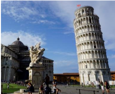
Fig. 7: The leaning tower of Pisa
